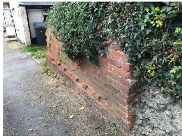
Photograph 10: Brick wall on developers' land
